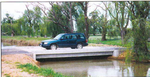
A typical 8 metre span double lane irrigation channel crossing. Techniques have been refined such that these simple bridges can be constructed in 3 to 4 days, including footings.
