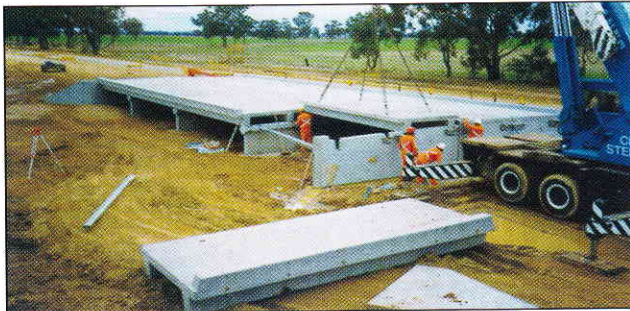
Semi-skilled workers with no previous experience assembled this Bridgette structure in 3 1/2 days. Cheaper than a conventional culvert the 7 metre spans are less prone to debris accumulation.
