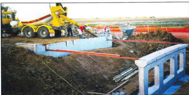
Temporary struts hold walls in place while bases are grouted. Apertures in walls reduce weight for transport and handling.
