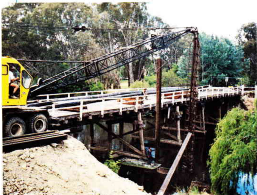
Above: 310UC97 steel piles driven from the riverbank.
