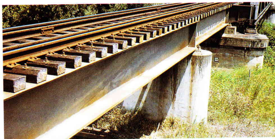
Stewarts River Rail Bridge - built to last.
