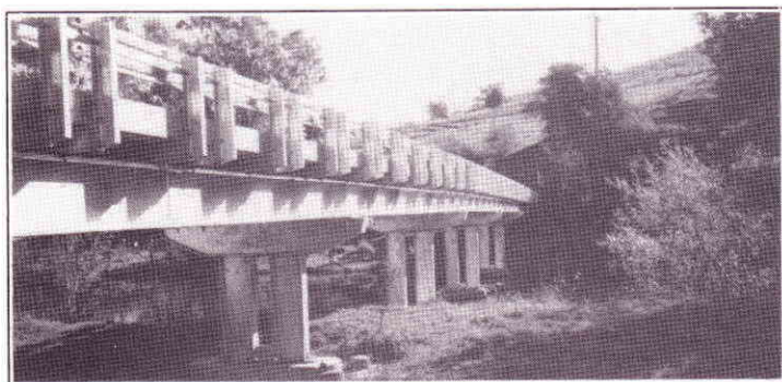
This bridge near Alexandra is supported on the timber piles of its predecessor. Although badly deteriorated above the piles were like new below. Capping them with concrete to support prefabricated galvanised steel piers and renewing the deck with Quickdek slabs enabled the bridge to be completely rehabilitated in a short time at low cost.
