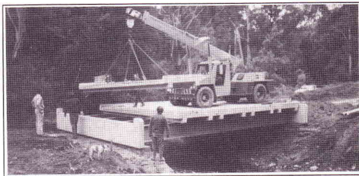
Superstructure "Kits" such as this, comprising steel girders, Quickdek slabs & matching fender walls, have saved time and cost of construction of new bridges such as this one on a forest access road near Myrtleford, and also for rehabilitation of old bridges.
