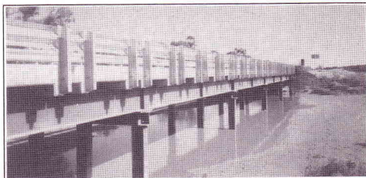
167km west of Bourke, this bridge has six spans totalling 54 metres overall length, comprising driven steel piles, steel girders and Quickdek slabs. The entire bridge "kit" together with pile driver and other construction equipment was transported to site by road train. Construction was completed in just over 2 weeks of arrival on site.
