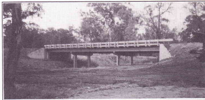
Quickdek slabs, steel piers & girders, and precast abutments enabled this bridge to be erected on pile cap footings in a matter of days. The abutments are in fact of reinforced earth design using "Tensar" geogrids embedded in the rear faces of the precast concrete walls.
