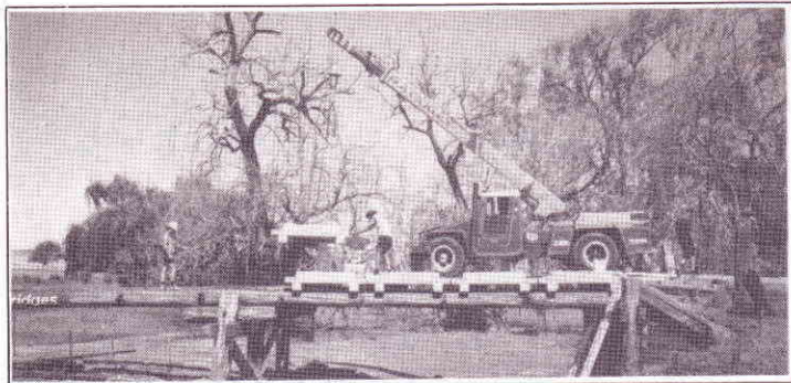
Dilapidated bridges such as this can be given a new lease of life when redecked with Quickdek slabs to distribute load across ALL girders is shown here by the crane which, with its load, weighs nearly 20 tonnes.
