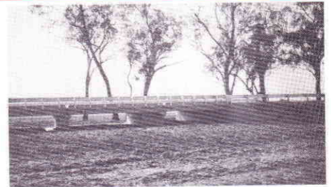
Bridgette planks have a shallow depth, similar to a conventional culvert, but the clear span is far greater. Waterway area is maximised, obstruction by debris is minimised.
